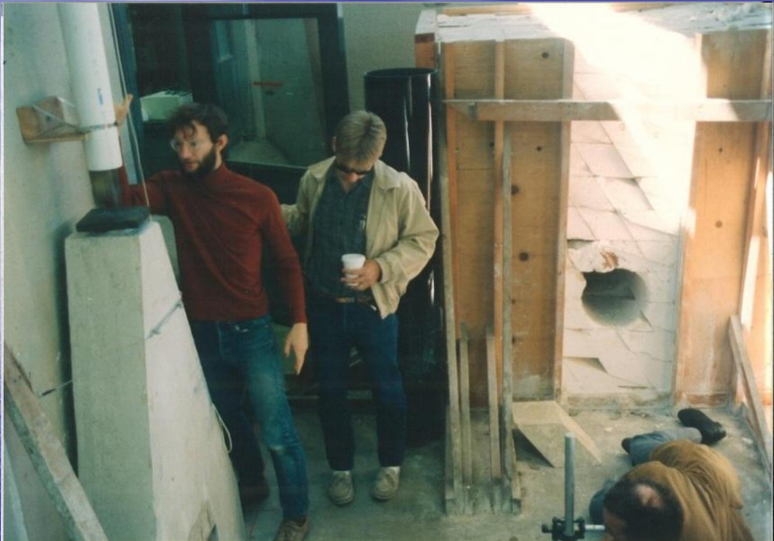
During his last decade at Berkeley, Dick's physical models became increasingly sophisticated. Anders Bro's PhD thesis was 6 foot cube model of three mutually orthogonal joint suites, through which he excavated a tunnel, shown at upper right.
