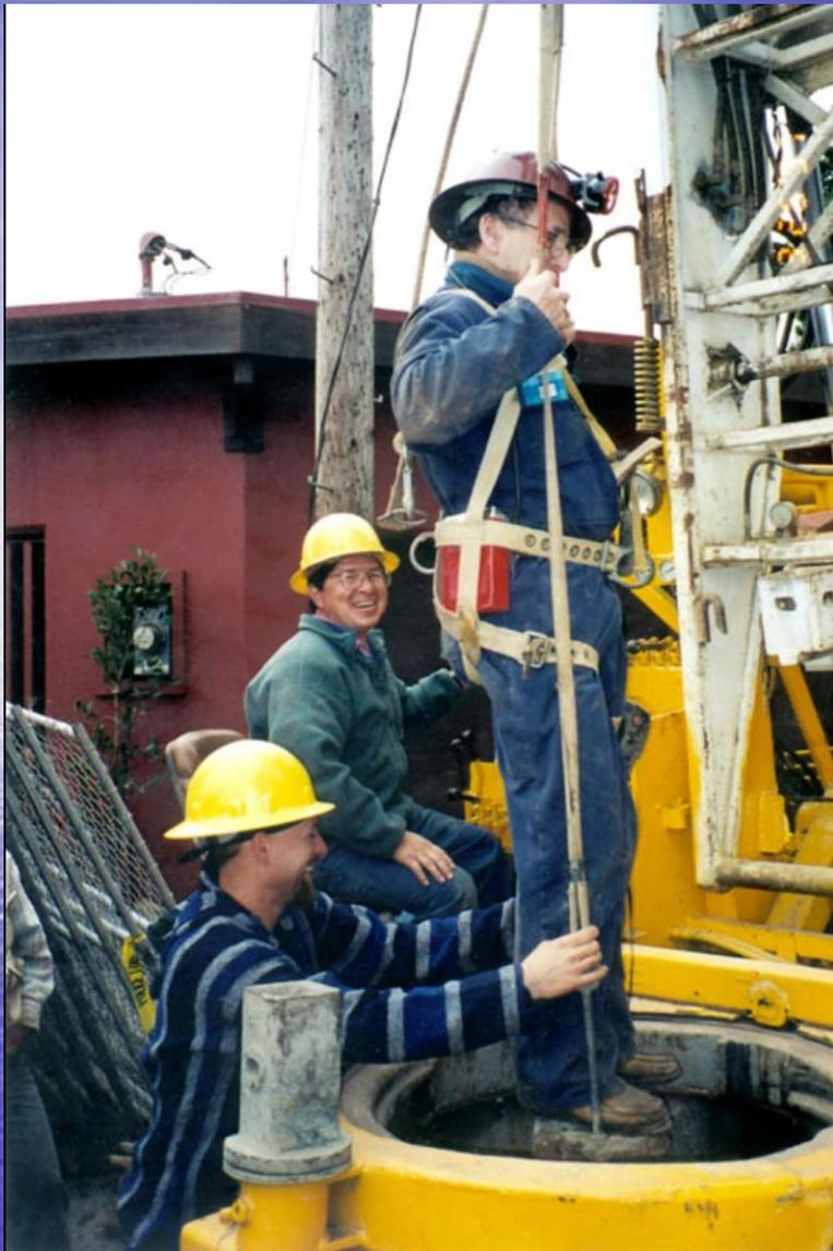
Dropping down bucket auger hole at Knockash Hill rock slide in San Francisco
